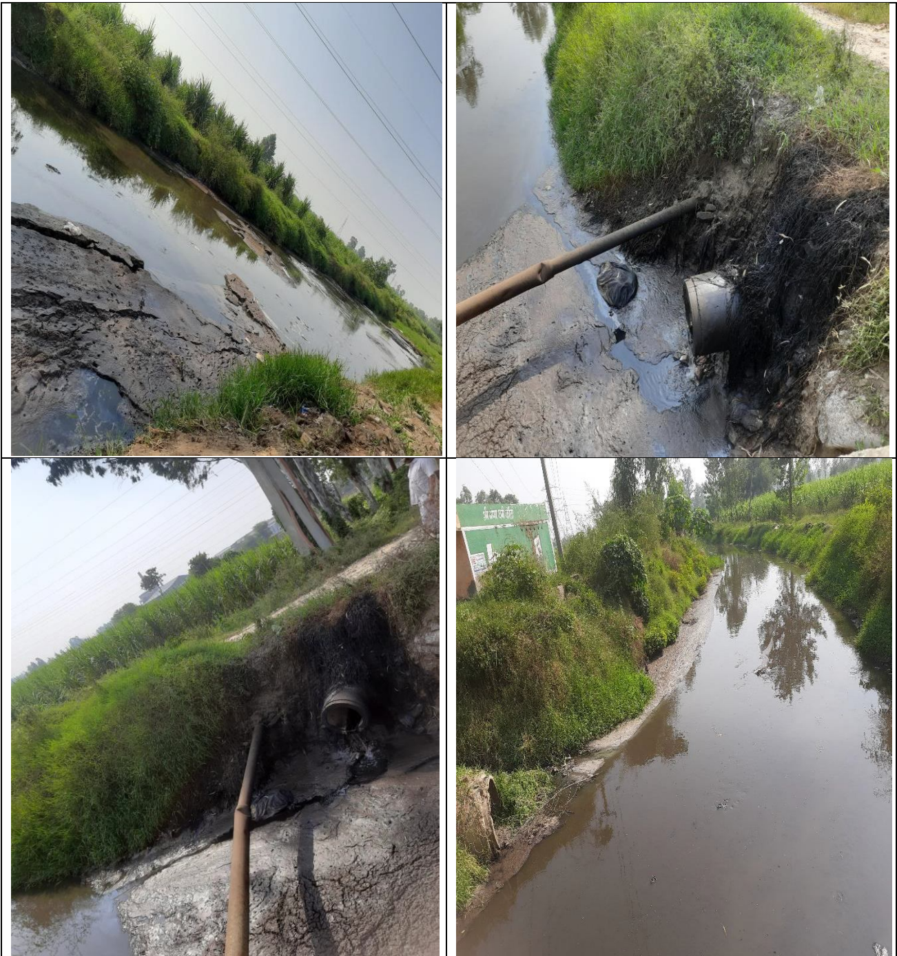
Dhandhera drain, Muzaffarnagar
